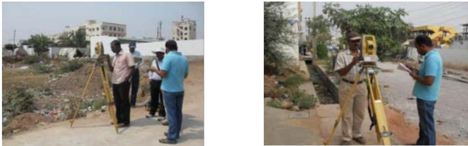
**Fig. 5. Traverse of the Gandhi Nagar Slum by Total Station**
